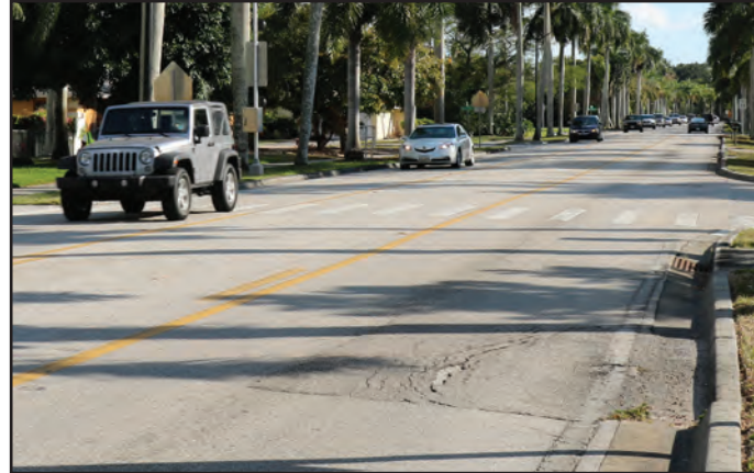
Example of existing storm drain pipe crossing to be improved.
